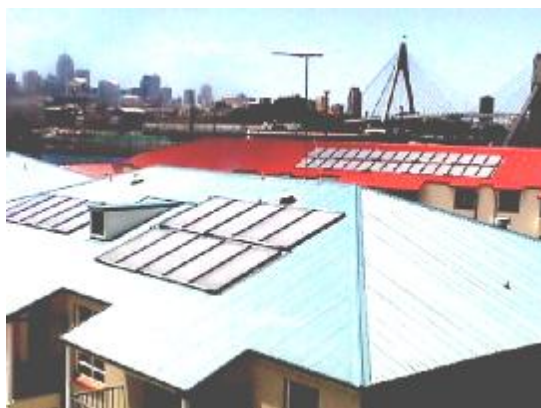
Centralised solar water heating on new housing at White Bay, Rozelle
